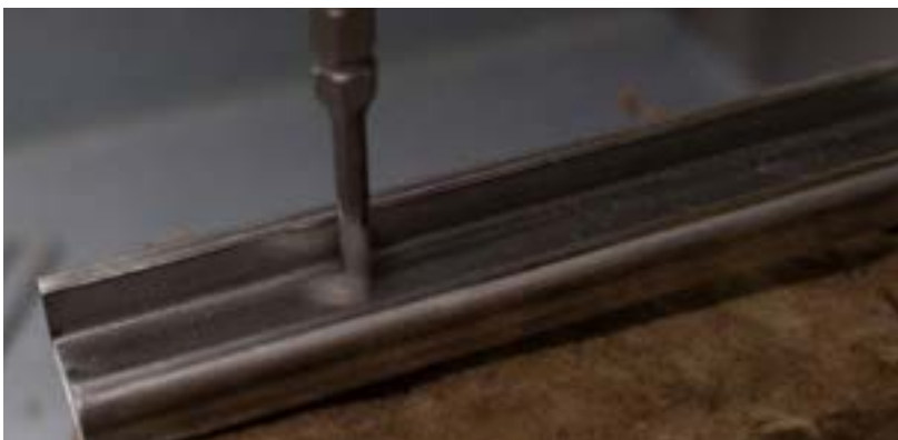
Figure11 – Drilling of pilot hole
