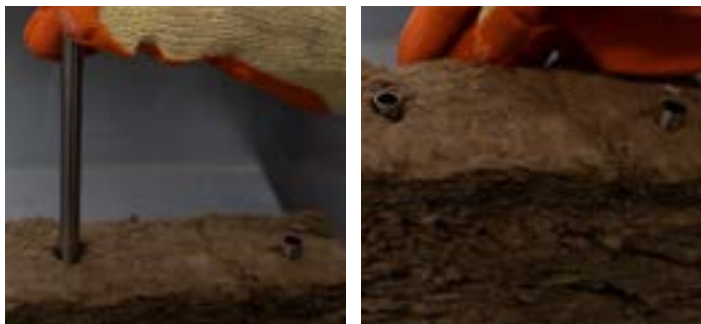
Figure 08 – Installation of anti-compression sleeves
