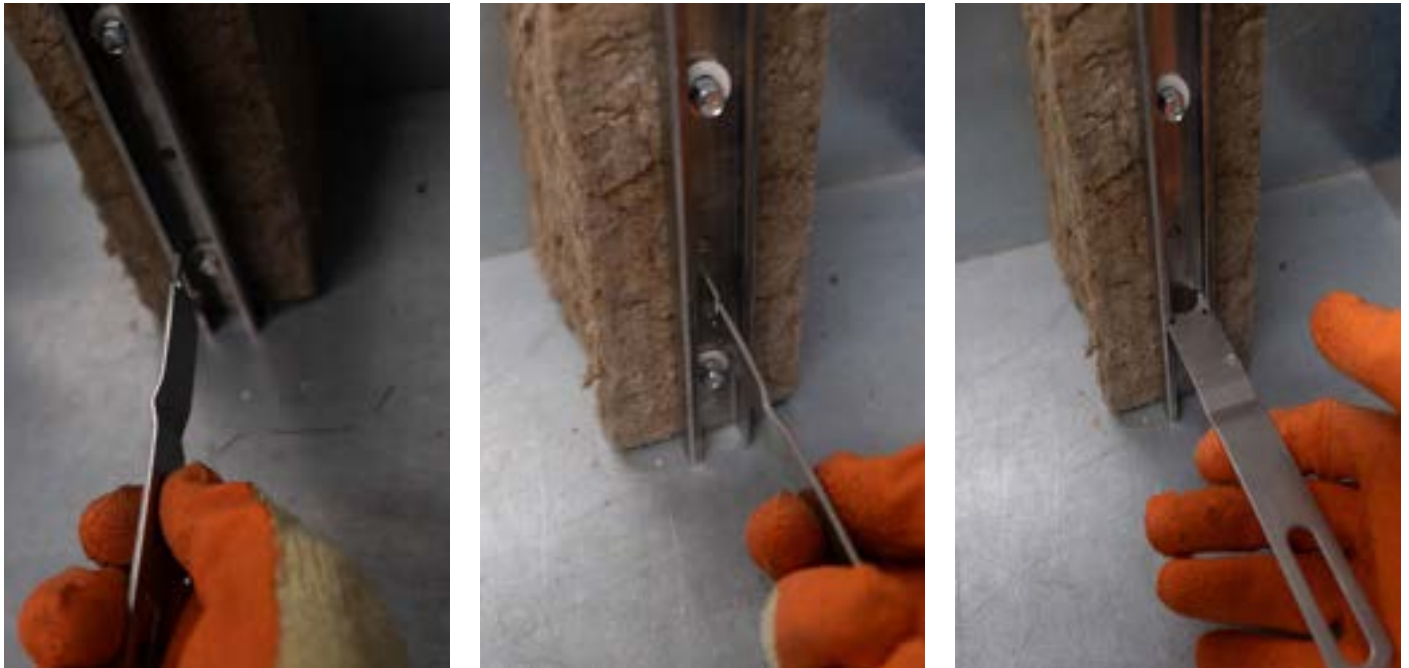
Figure 13 – Installation of wall-ties into retention channel
